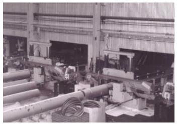
Figure 1. An overview of the Saw Shop showing the cutting of ingots into wheel blanks.
